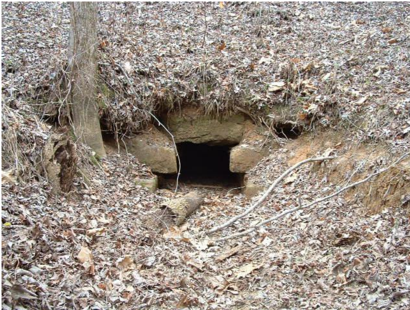
Figure A-10 This is the north side entrance into tunnel 4, this tunnel is created of concrete blocks and is approximately 0.5m.x0.75m.
