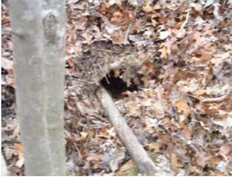
Figure A-7 this is the south side of tunnel 3, the small metal pipe is barely visible
