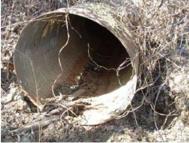
Figure A-3 This is the south entrance of the tunnel
