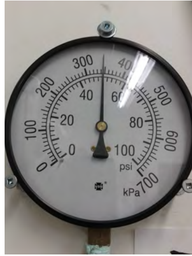
(b) The pressure gauge for the cooling water of e-gun/thermal deposition system.
