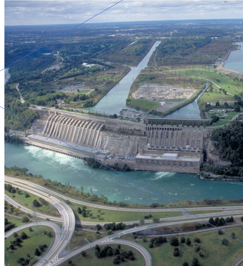
Sir Adam Beck Hydroelectric Power Station (Ontario)
