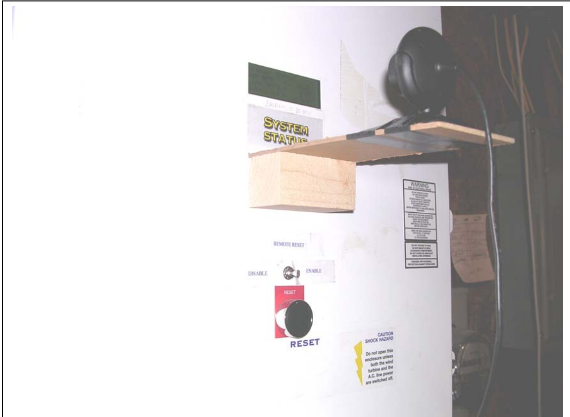
Figure 2: A cheap Web-Cam is mounted on a wooden shelf (1.5" by 7") attached to a wooden block (1.5" x 1.5" x 3"). Two 1/8" holes were drilled into the GridTek10 door to pass two wood screws thru the sheet metal to attach the wooden block.
