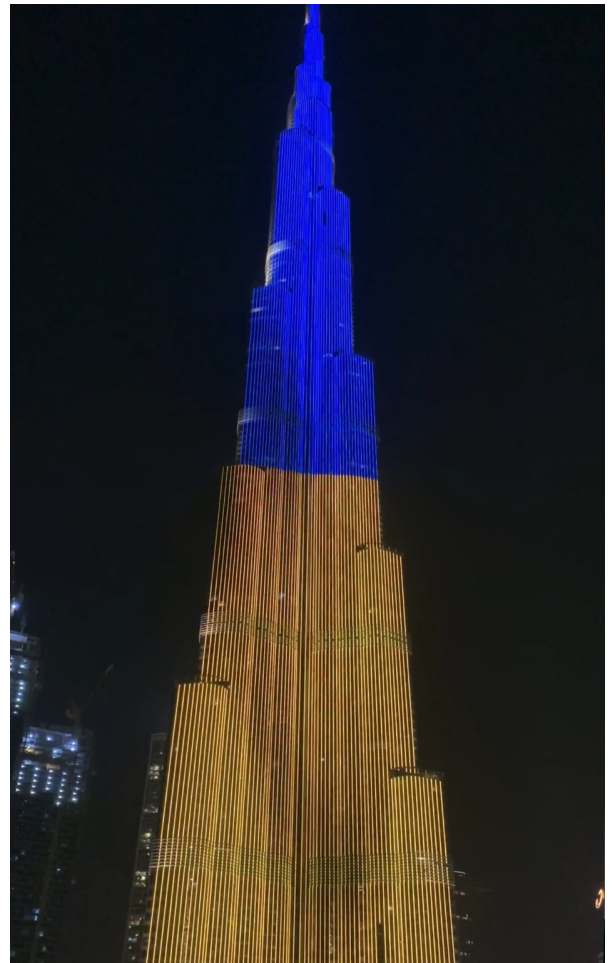
Dubai, UAE. Source: https://shorturl.at/e36Q6
