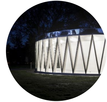
PAVILION BUILDING - ARCHITECTURALLY INTERGRATED LUMINAIRES
