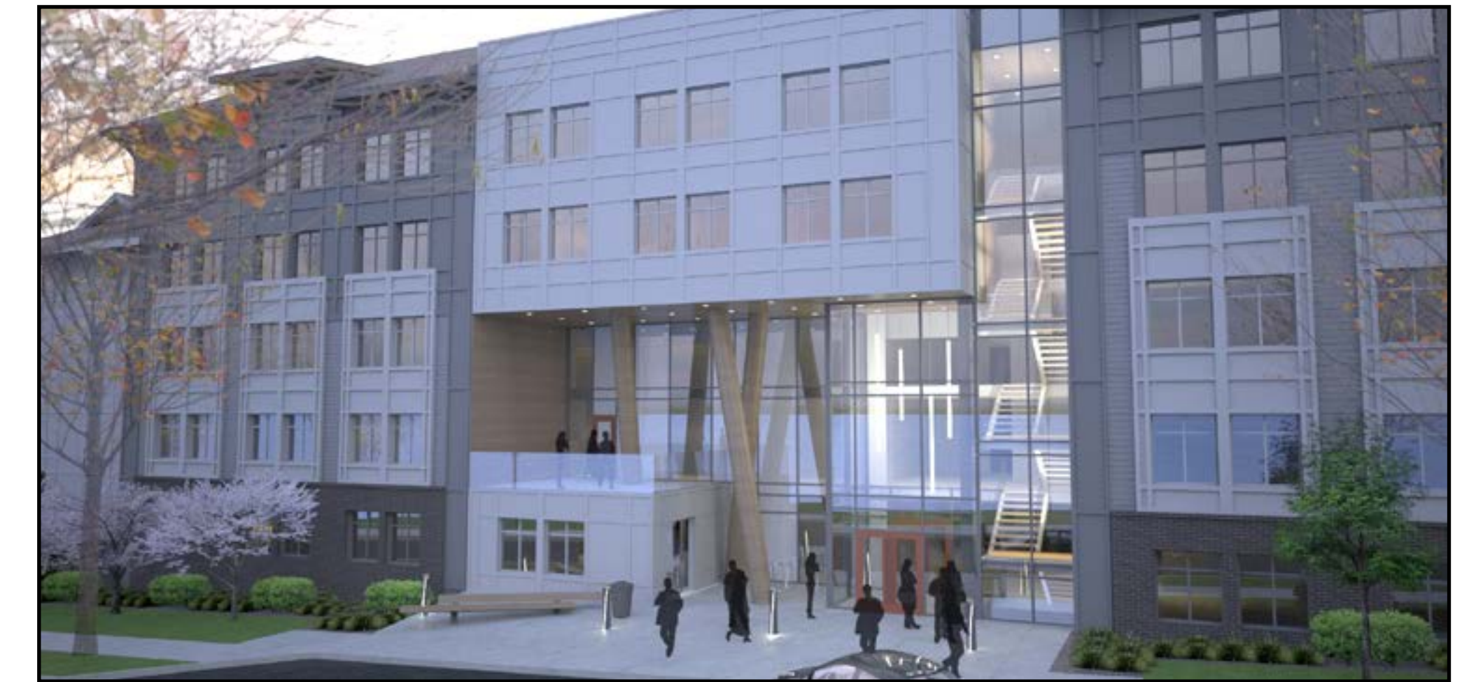
Main entry on 111 Street.
