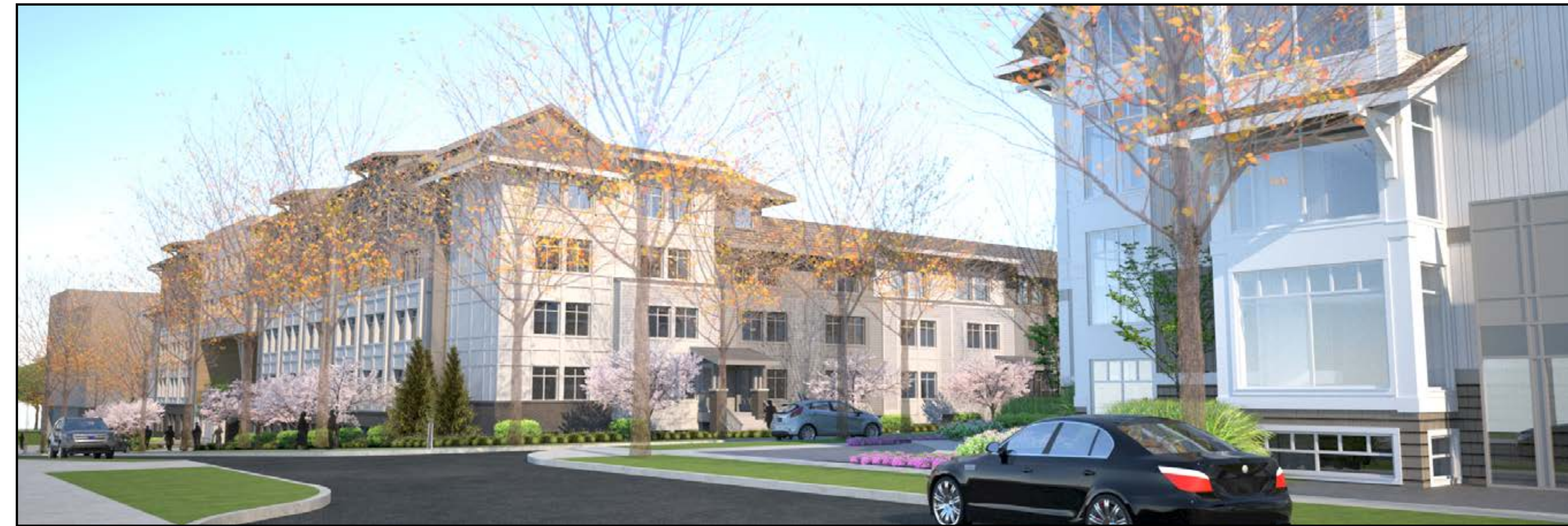
View northeast from 111 Street (Pinecrest House to south).
