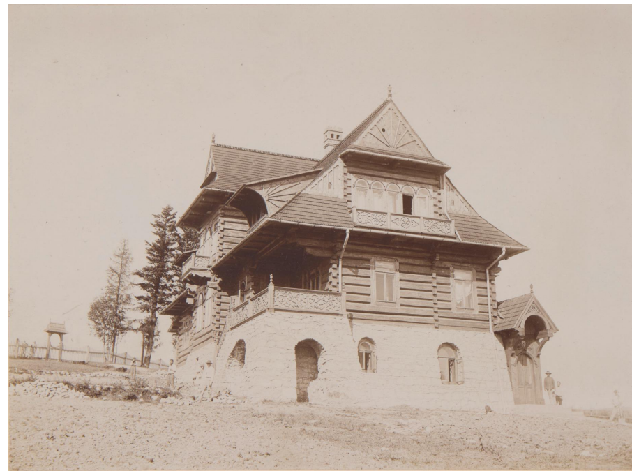
Villa „Under Jedla” in Zakopane, designed by Stanisław Witkiewicz (PL), owned by the Pawlikowski family, circa 1898-1905, National Museum in Cracow
