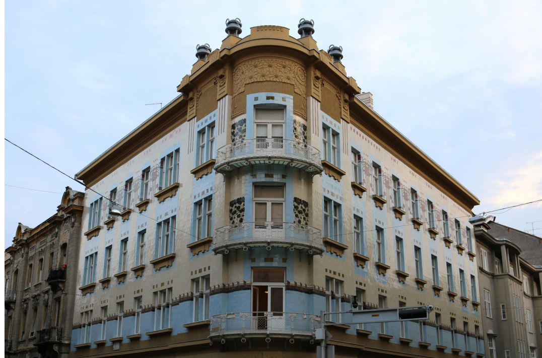
Kallina House in Zagreb, designed by Vjekoslav Bastl (HR), authors' private archive
