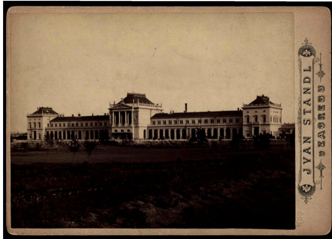
Main Railway Station in Zagreb, photo by Ivan Standl (HR), 1893, National and University Library in Zagreb
