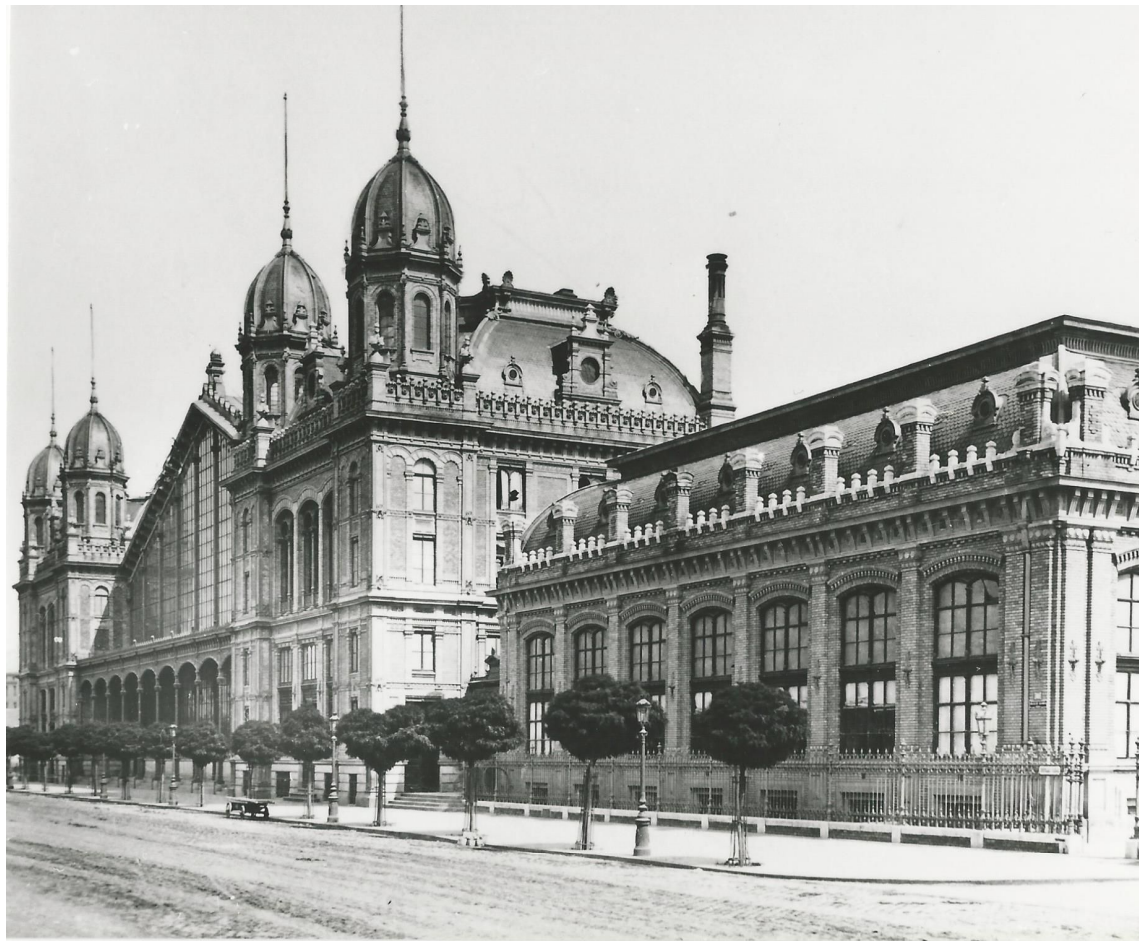
Western Railway Station (Nyugati) in Budapest, designed by Eiffel Company, early 20th century, Hungarian Museum of Trade and
