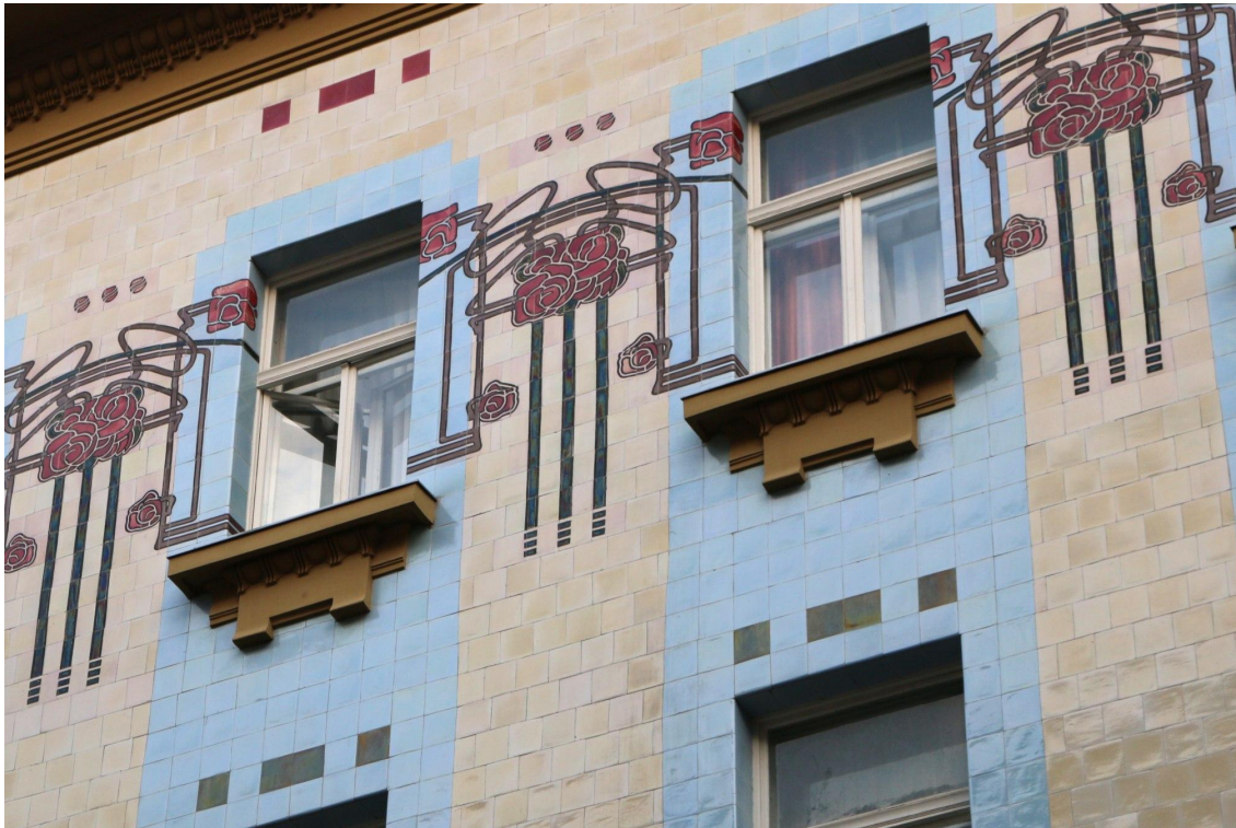
Kallina House in Zagreb, designed by Vjekoslav Bastl (HR), authors' private archive
